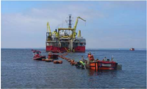
Use float over – vessel stays in deeper waters
